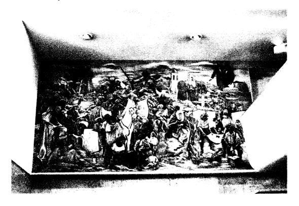
The west wall mural is by Charles Alston, 1949, signed bottom right. The condition is also very good. Surface percussion indicates some voids. The marouflage adhesive is likely the same as on the east wall. A fresh peel test along the left side of the door reveals relatively easy detachment from the wall. The canvas is not wrapped and is cut flush to the door edge.
